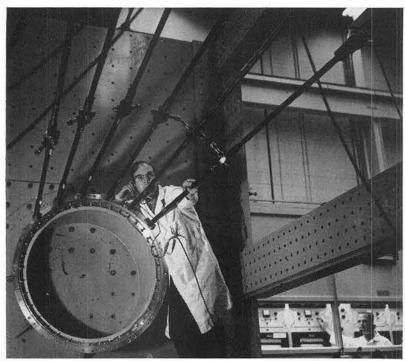
PARACHUTE FIXTURE, about to be tested, is mounted inside one of the steel frames in Bldg. 864. Howard Nunez checks the six pull rods which will exert force on the fixture. Bill Putnam, lower right, is in the control room where automatic equipment can run test.
